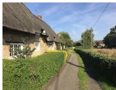
Footway separated from carriageway
